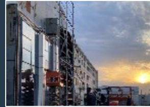
Curtain Wall Test Lab Shanghai, China
