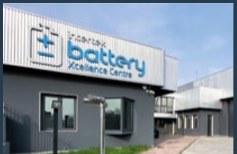
Battery Xcellence Centre Mestre, Italy
