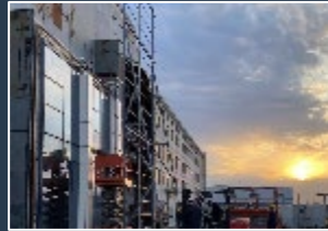
Curtain Wall Test Lab Shanghai, China
